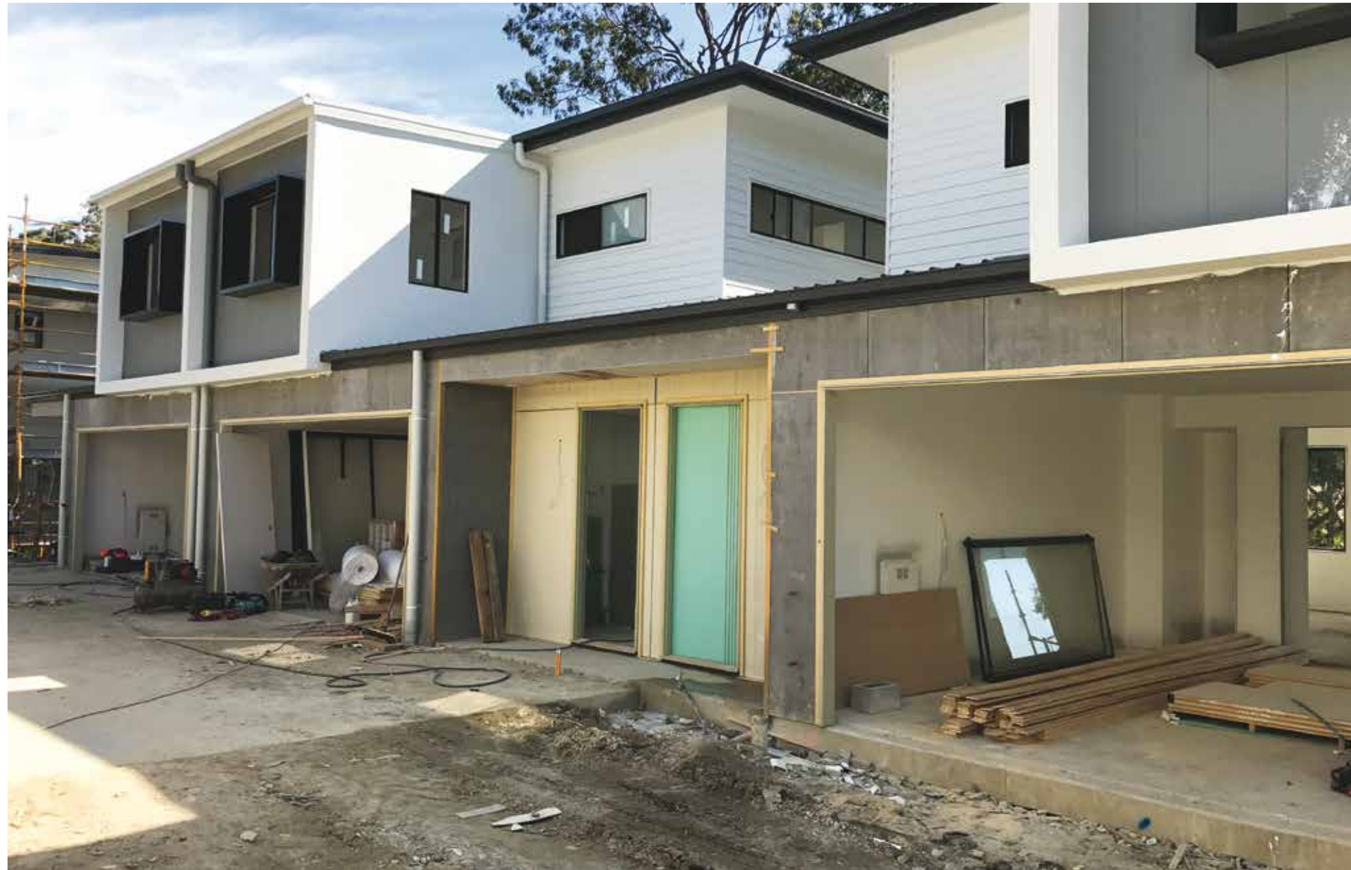
External painting commenced for town houses 1 – 7. Rendering and wall coating commenced for town houses 3 – 7, as well as the construction of internal partitioning. Cladding for town house 11 was also completed and a start made on the rendering and wall coating process.
