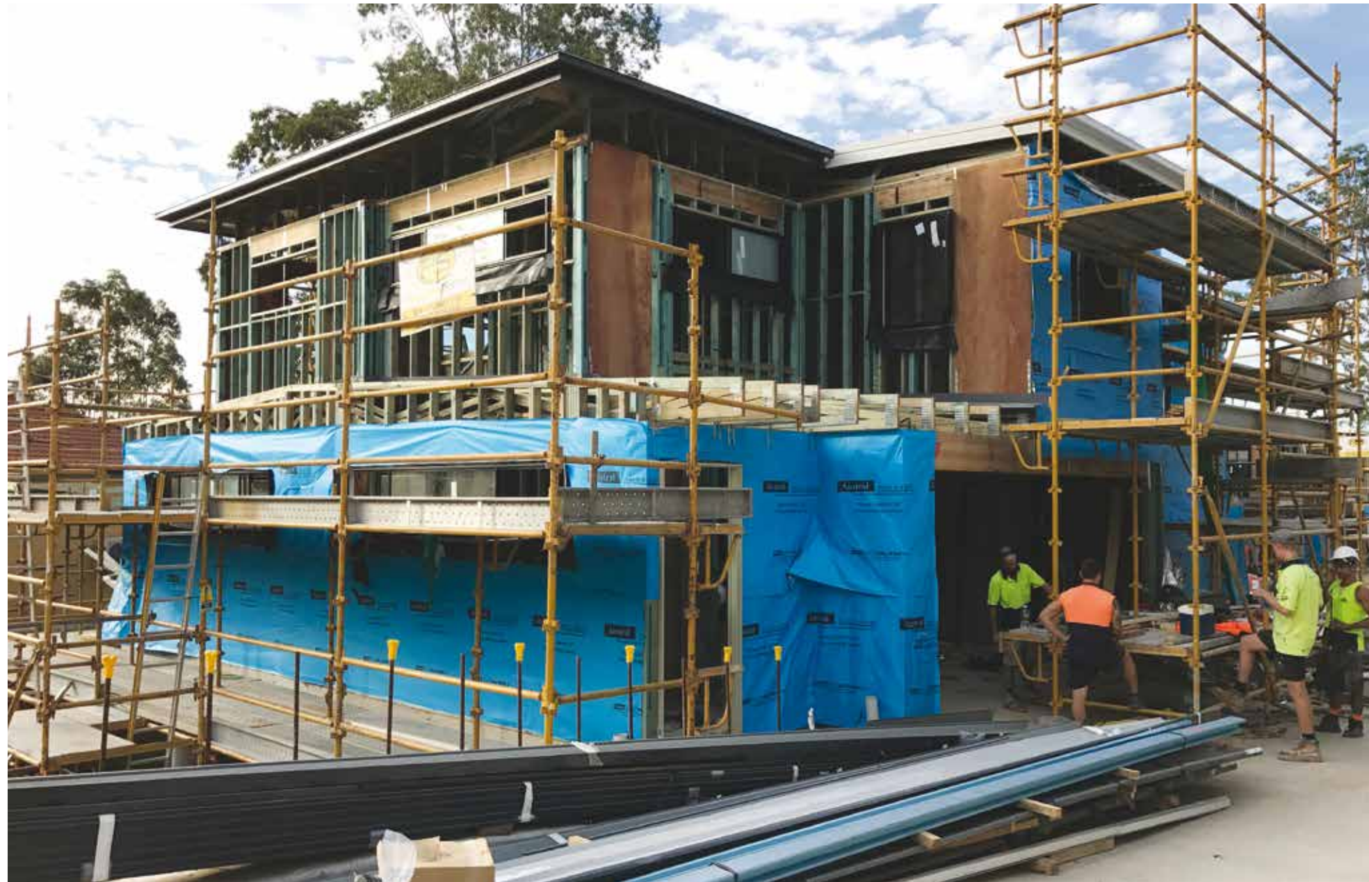
With the completion of the suspended slab upon which town houses 1 and 2 sit, work could commence on the framing of walls and floors. In town houses 8 – 11, building pads were cut, ready for footings and slabs to be poured. The external walls of town houses 12 – 18 had cladding erected, while internal framing and service rough-ins were completed for town houses 12 – 14 and are underway in 15 – 18.
