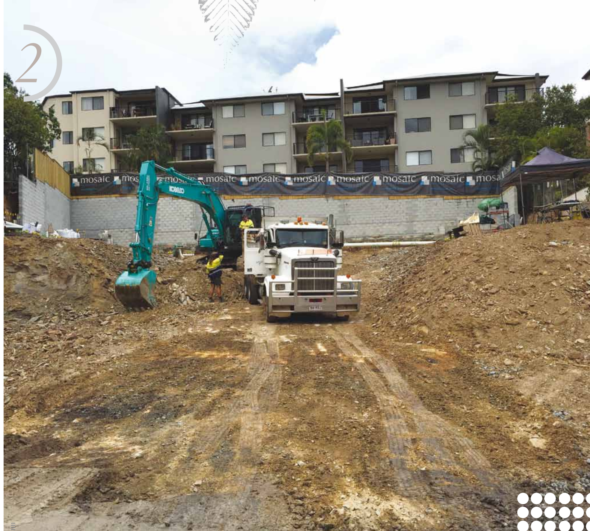
CONSTRUCTION UPDATE / MARCH 2016 /
