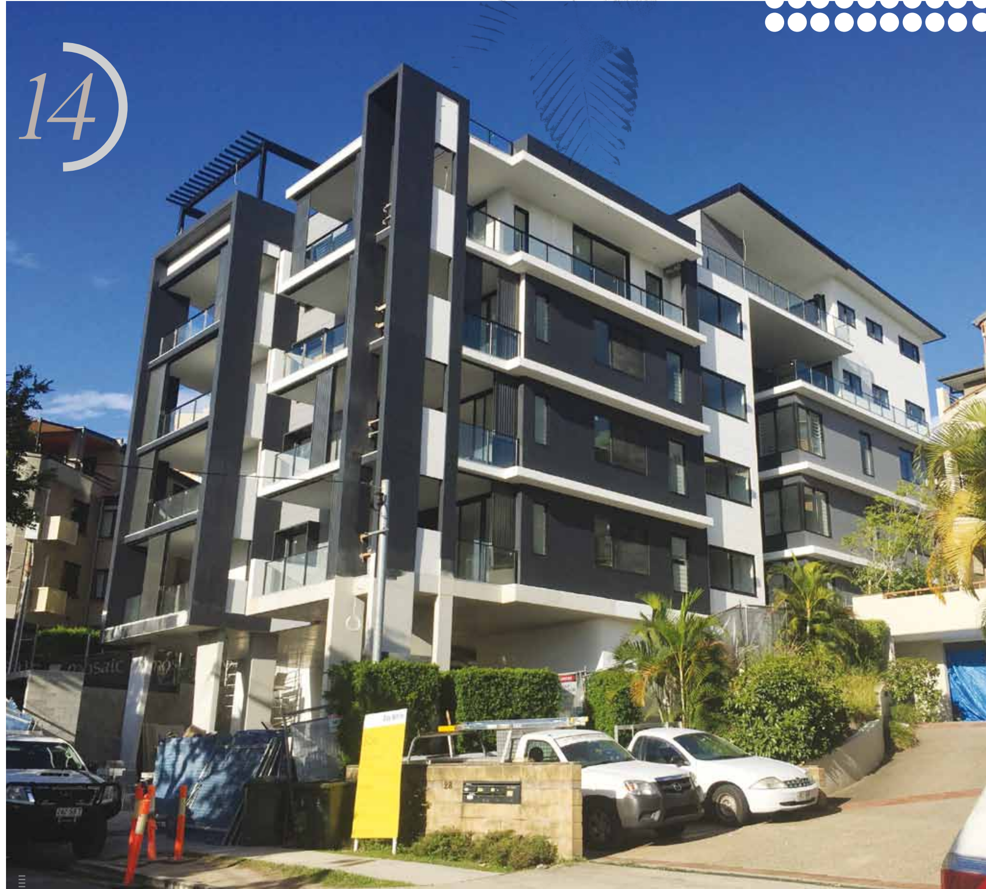
CONSTRUCTION UPDATE / MARCH 2017 /
