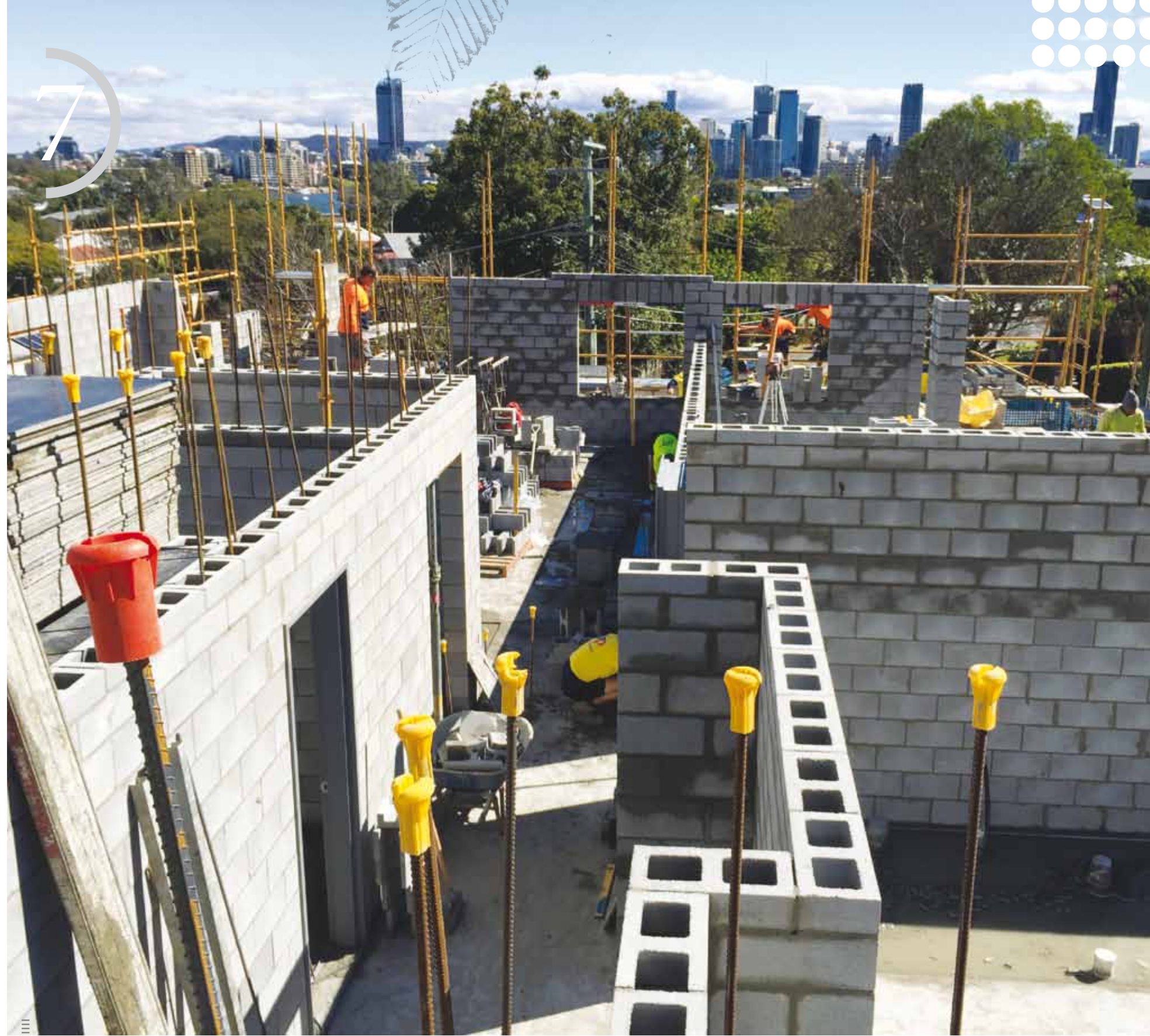
CONSTRUCTION UPDATE / AUGUST 2016 /
