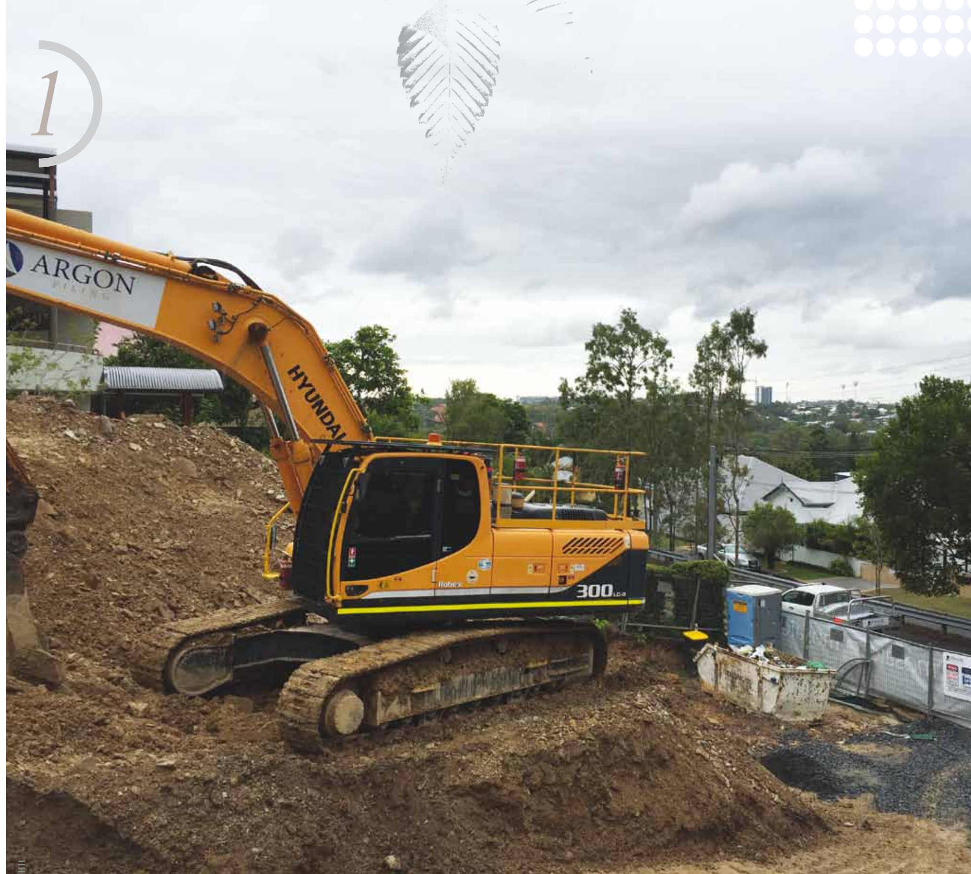
CONSTRUCTION UPDATE / FEBRUARY 2016 /
