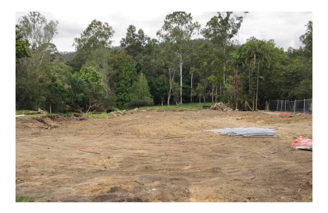
With Operational Works and Building Approvals in place, the existing dwelling was demolished and the site perimeter fencing set-up around the waterway corridor at the rear of the site which will be further rehabilitated towards the end of the project.
