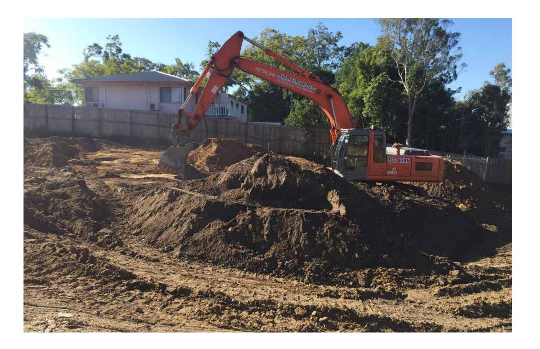
With the site office mobilised, earthworks and excavation commenced. The temporary erosion and sediment control basin was established, which will capture stormwater run-off from the site during the construction phase and ensure that stormwater discharge to the waterway is of appropriate quality.
