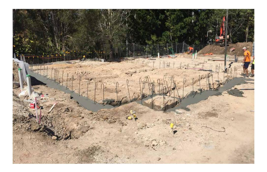
The building pads for town houses 10 through to 14 had underground services roughed in and bedding material applied and compacted before the slab was formed up and poured, marking the completion of the first of the concrete slabs.
