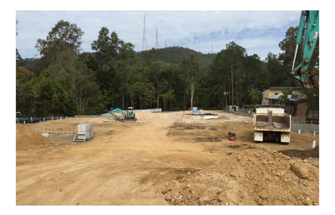
Although the final earthworks around town houses 1 - 4 were still to be finalised, building pads for the house slabs of town houses 5 through to 20 were benched out ready for the final trim – the site is taking shape.
