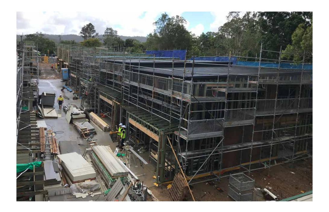
Despite persistent wet weather, scaffolding for town houses 8 to 17 was installed, allowing external façade works to commence. With fascia gutters and roofing installed for town houses 10 to 17, work could continue inside despite the rain.
