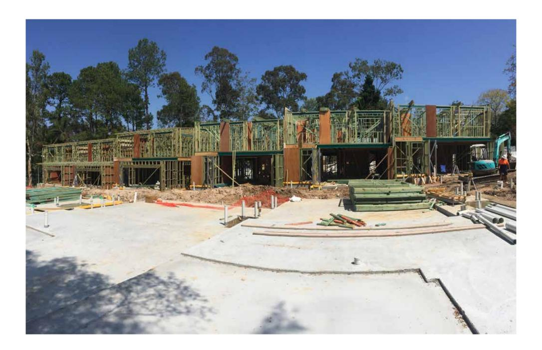
Slabs were poured for most of the town houses, with many also framed or with frames ready to be erected. Town houses 12 to 17 had upper level flooring installed and plumbing services roughed-in ready for roof installation, while the strip footings of town houses 18 to 20 was poured.
