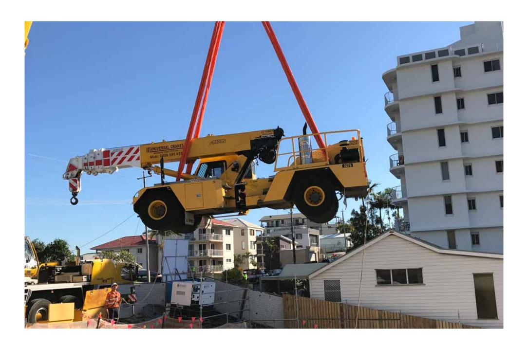
With the bulk excavation complete, two 12-tonne stormwater detention tanks were installed, which required a 130-tonne crane to lift a 35-tonne crane and a 25-tonne crane into the excavated site – a very difficult manoeuvre.
