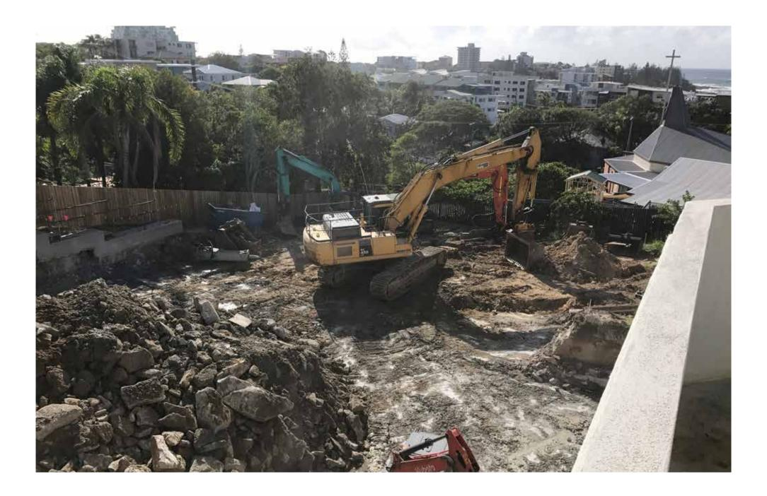
Even though the difficult conditions required a 35-tonne excavator equipped with a rock breaker on site, the soldier piles around the perimeter of the basement carpark were completed as well as the capping beam which distributes the loads from the building above down into the solider piles.
