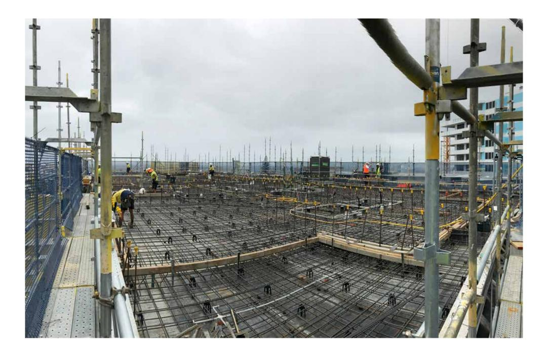
The building moved steadily upwards to Level 3, with formwork, steel reinforcement and service rough-ins followed by the pouring of the suspended slab.
