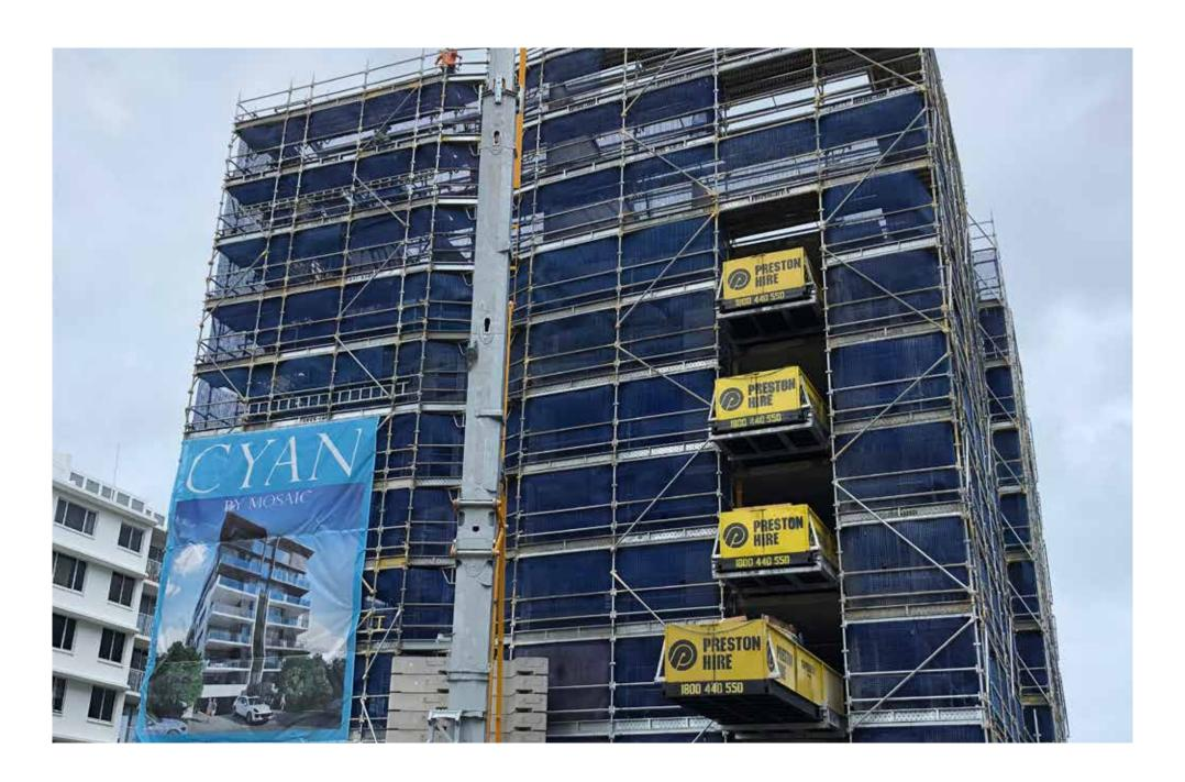
The building reached its full height with the pouring of the final slab. As roof framing on the final level neared completion and blockwork progressed on the Penthouse Level, the glazing, framing and sheeting of apartments reached Level 6.
