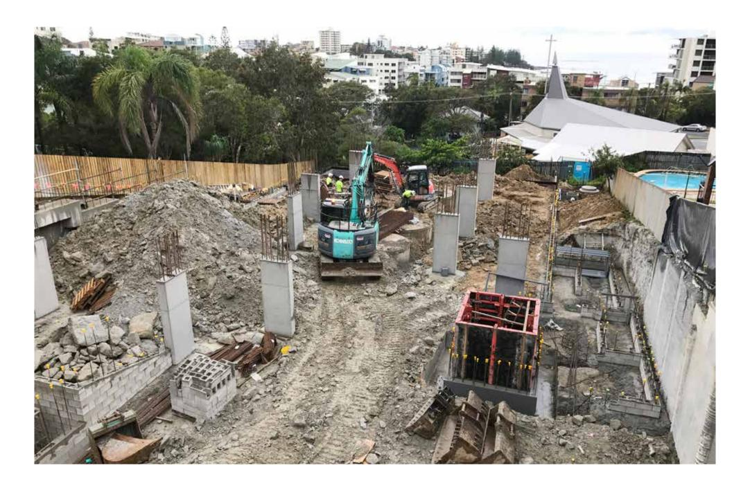
A major milestone was reached with the pouring of the first slab, the 'Basement Level 2' slab-on-ground, which will now provide a solid area of hardstand to work off as the building begins to move upwards out of the ground.
