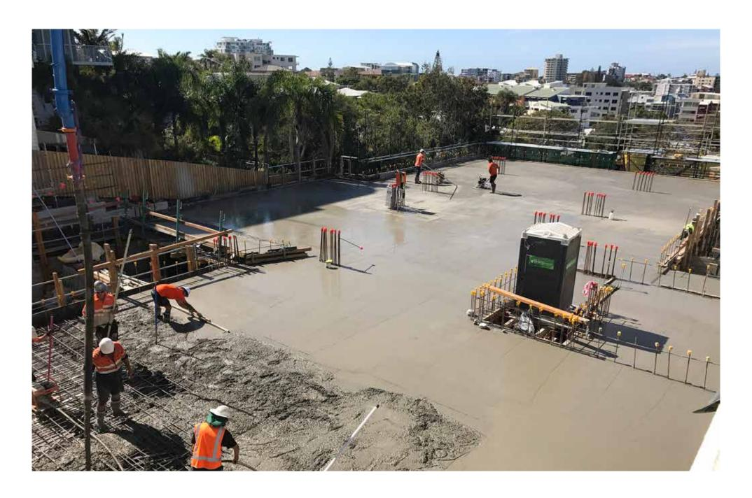
With the first of the eight suspended slabs (Basement Level 1) successfully poured, structural works continued on Basement Level 1 with the blockwork walls, service penetrations and fire door frames all completed.
